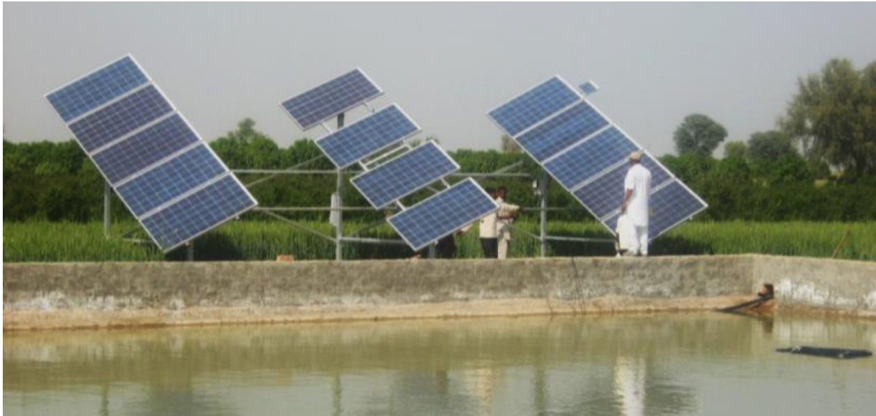
Solar pump for drip irrigation with Floating platform (Ganganagar, Rajasthan )
