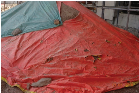
Construction material with a tendency to get airborne are covered
