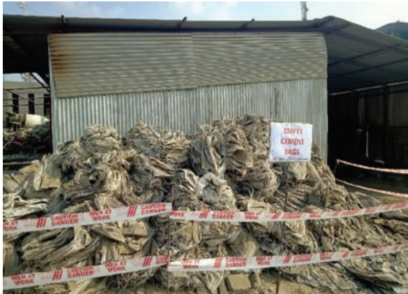
(5) Disposal of C&D waste- segregation of construction materials and waste
