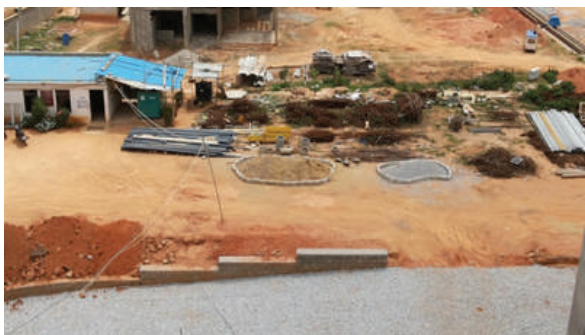
(3) Construction Phase- Soil erosion channels and sedimentation pits constructed around the sites
