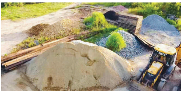
(7) Building of stockpile
