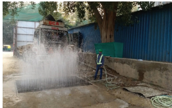
(3) Vehicle waiting area and hard standings- Use of wheel washing and anti-fog guns at construction sites
