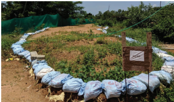
(3) Construction Phase- Soil erosion channels and sedimentation pits constructed around the sites
