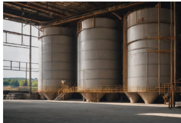
(4) Storage of cement and other similar materials- Should be stored in silos having ventilation system fitted with particle filters
