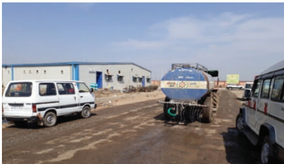
(1) Haul roads and traffic routes- sprinkling water
