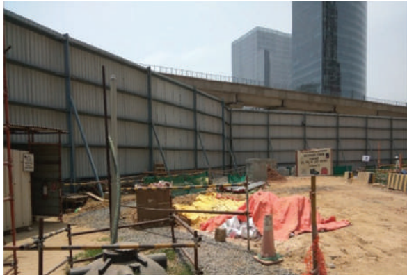
(1) 3 metre high continuous barricading
