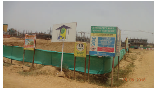
(2) Site Traffic- speed limit of vehicles on site to 10 km/h
