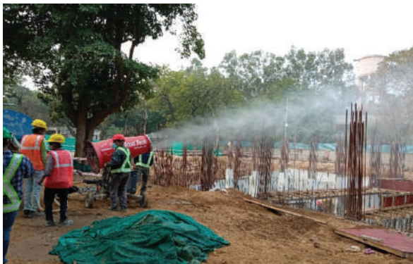
(3) Vehicle waiting area and hard standings- Use of wheel washing and anti-fog guns at construction sites
