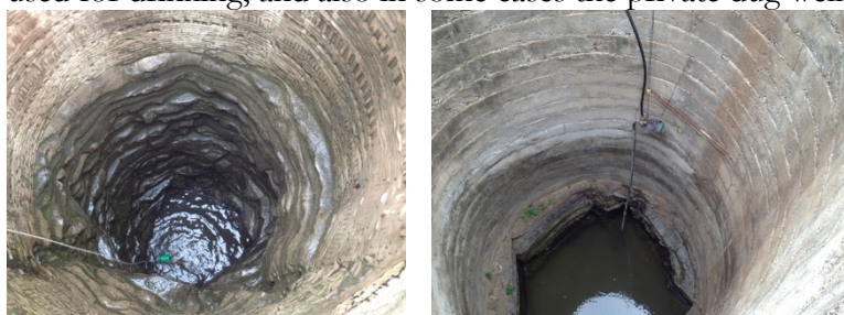
Figure 4. Open wells in Warudi village during September 2012
