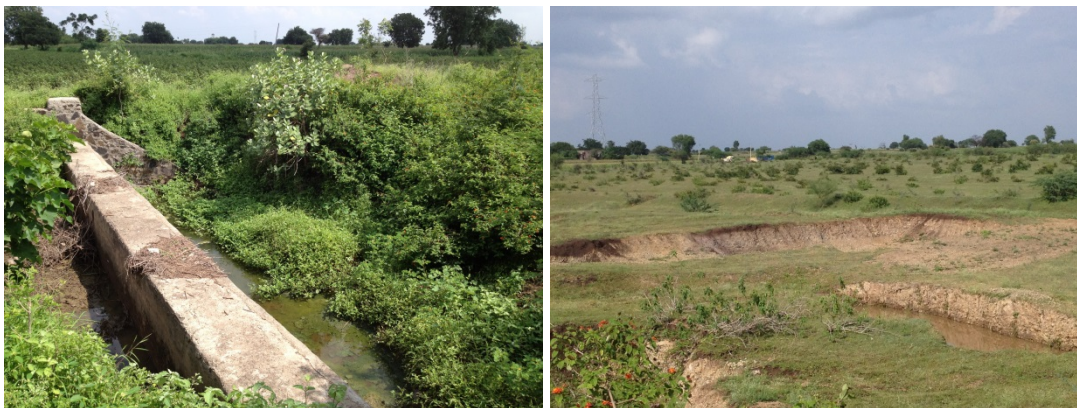
Figure 6. Watershed structures. 6a (left): a small check dam. 6b (right): percolation tank, Sep. 2012
