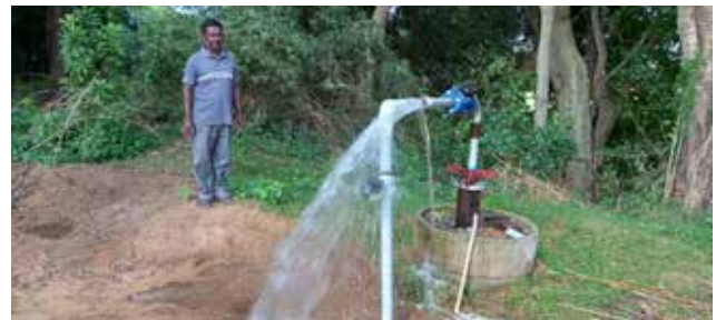
▶ Riverbank Filtration Well at Kapila River in Mysuru implemented for meeting drinking water supply
