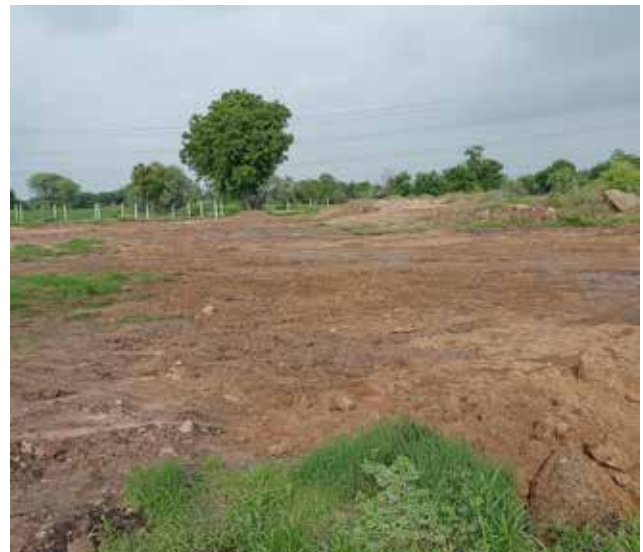
► After bioremediation of oil contaminated land
