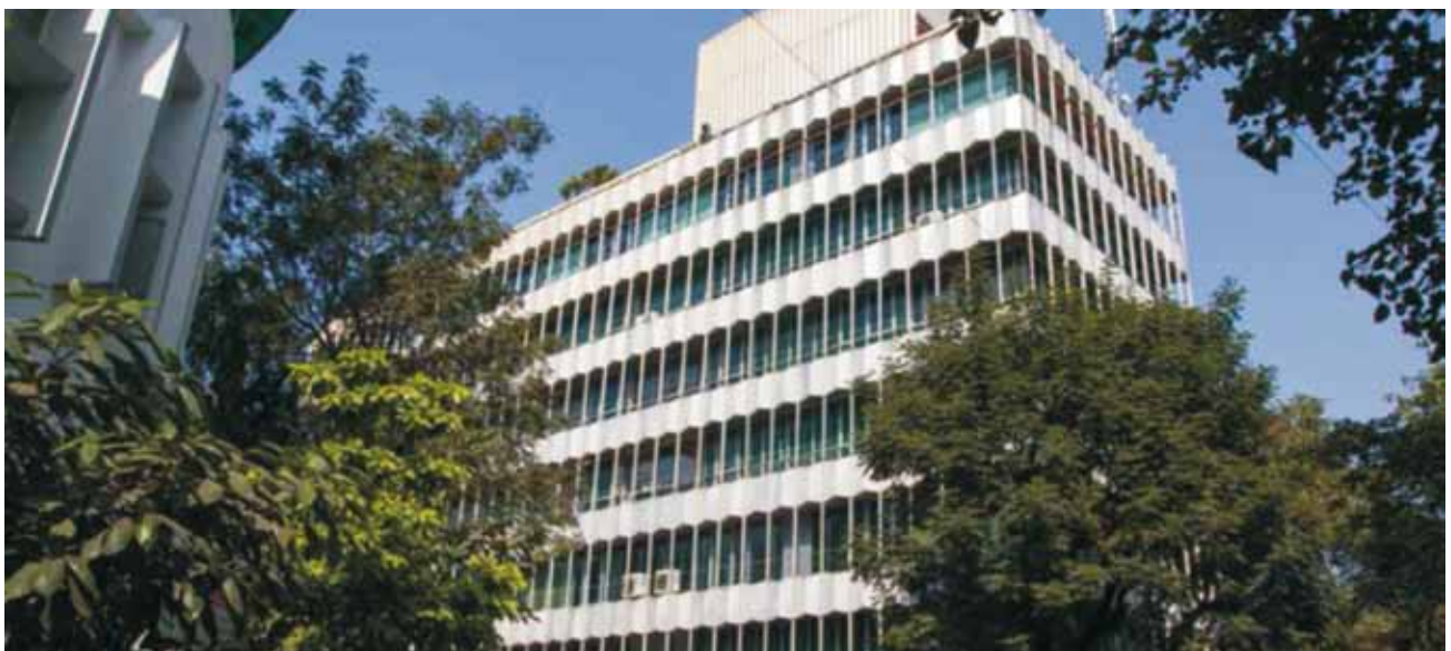
Figure 1 :Street View of Godrej Bhavan
