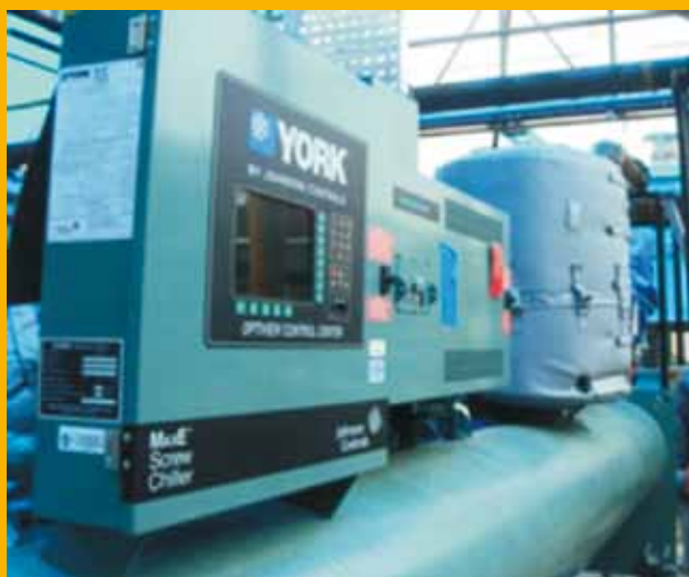
Figure 1: Replacement of Air Cooled Chiller to Recycled Water Cooled Chiller at the ITC Plant in Bangalore
