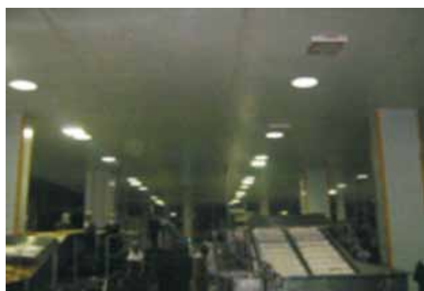
Figure 1: Sky pipe lighting at the Food Processing industry
