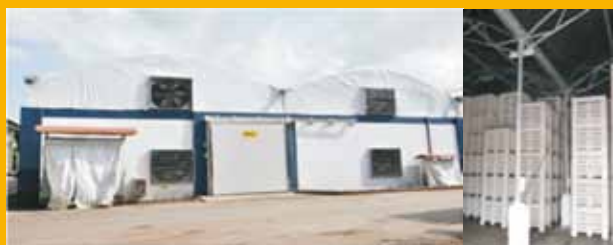
Figure 1: Evaporative Cooling Ripening Chamber at Food Park, Jain Valley, Shirsoli Road, Jalgaon
