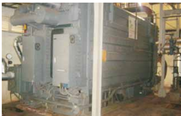
Figure 1: Vapor Absorption Machine based chillers at Food Park, Jain Valley, Shirsoli Road, Jalgaon
