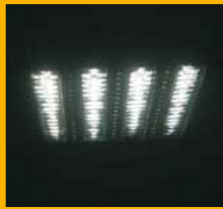
After with 4X14Watts T5 light fixture
