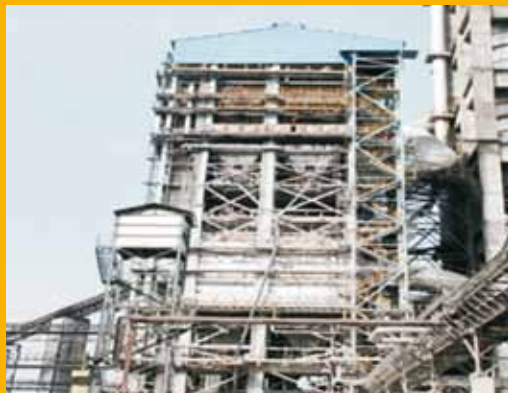
Figure 1: Installation of Waste Heat Recovery system to trap the waste heat from preheaters and Air Quenched Coolers (AQC) of Clinker manufacturing pyro process to trap the waste heat
