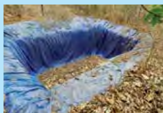
Tank for rain water harvesting- jal kund
