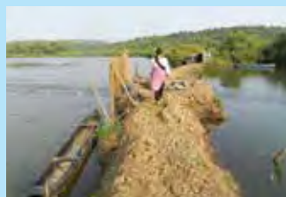
Bund, Sluice gate
