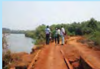
Candlim sluice gate
