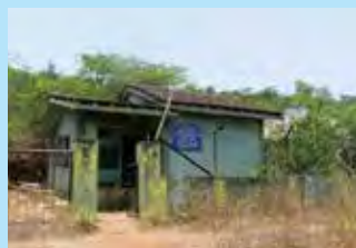
PWD water tank
