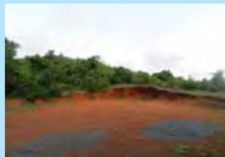
Excavation and levelling
