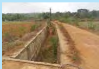
Storm water drain
