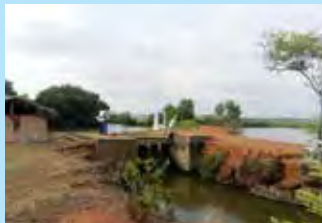
Manos/sluice gate and bundh/embankment
