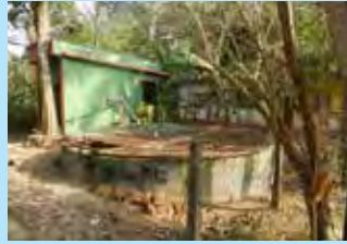
PWD water tank
