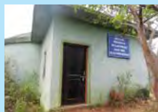
PWD water tank
