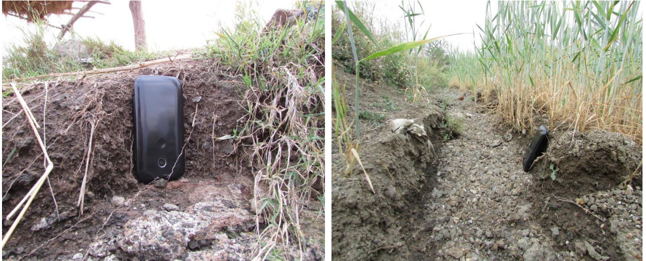
Photo 4.1 Land degradation resulting in production losses for farmers
